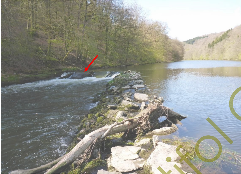
The Vanne des Moines dam, with a pass located along the right bank (often tricky to cross, strong current). Caution is required. It is possible to disembark on the right and carry your boat past the dam before re-entering the water, avoiding the descent by boat.
